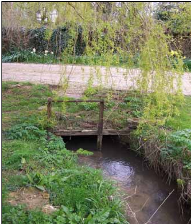
Coldwell Brook, driveway crossing to Coldwell House looking upstream
