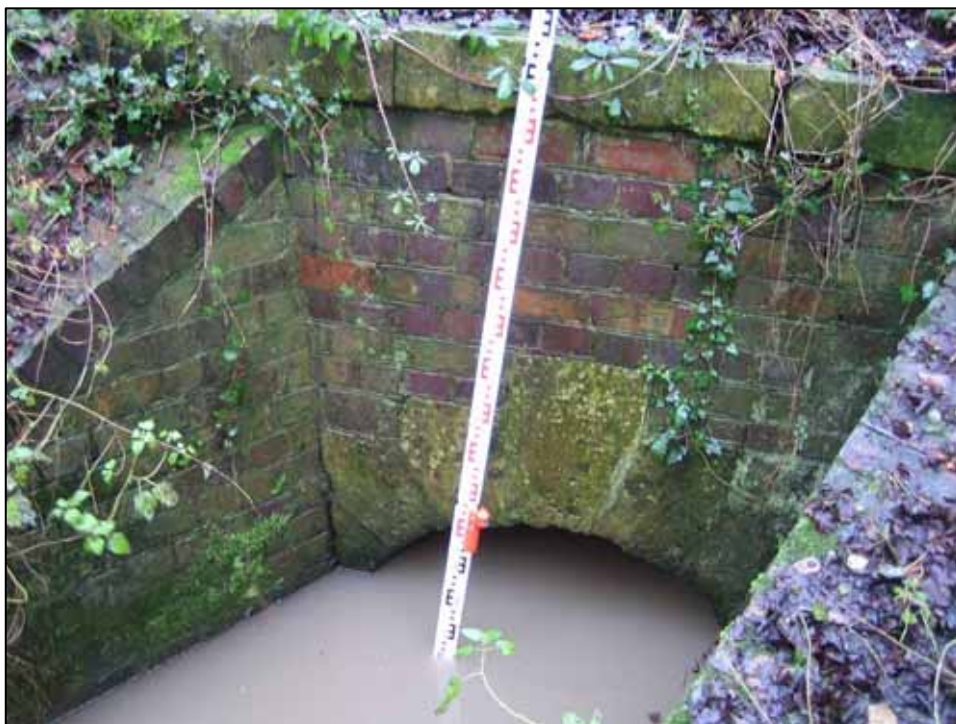
Downstream face of railway culvert – Shipton Road (EA Copyright)
