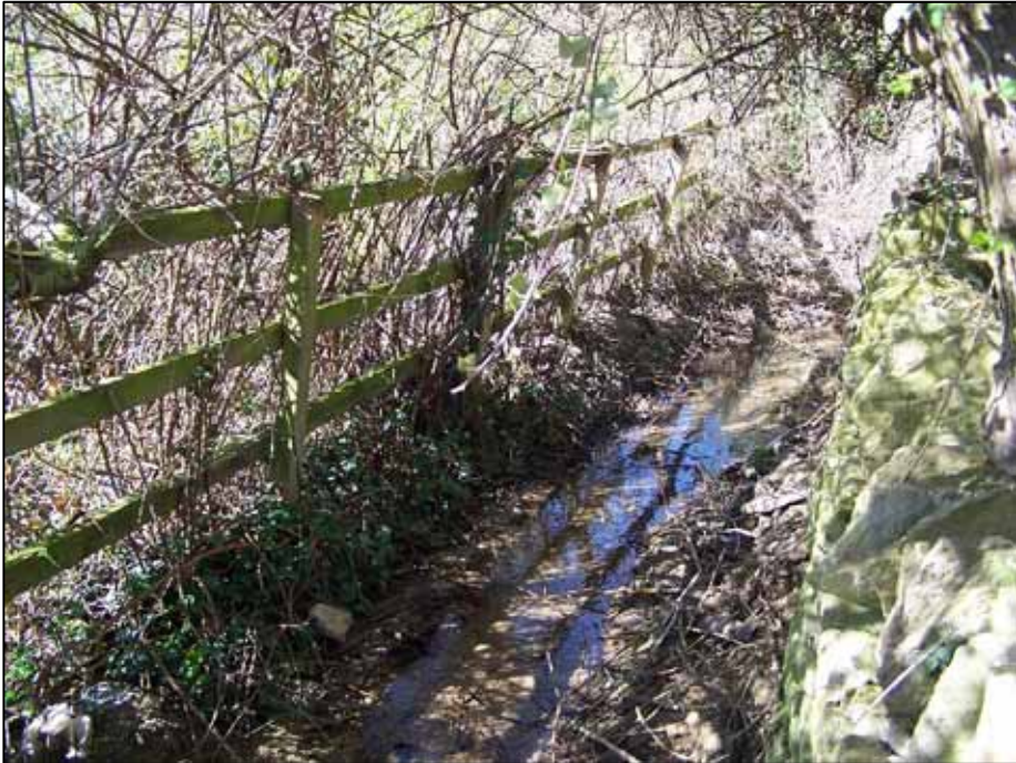
Downstream of stretch of watercourse at High Street, overgrown
