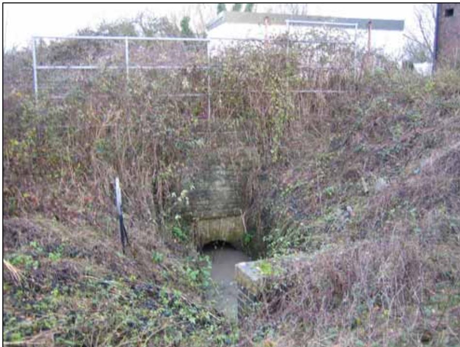
Upstream face of railway culvert – Shipton Road (EA Copyright)
