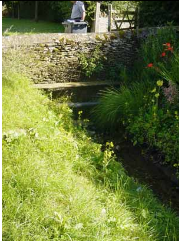
Upstream Entrance to 750mm Diameter Culvert North of Main Road.
