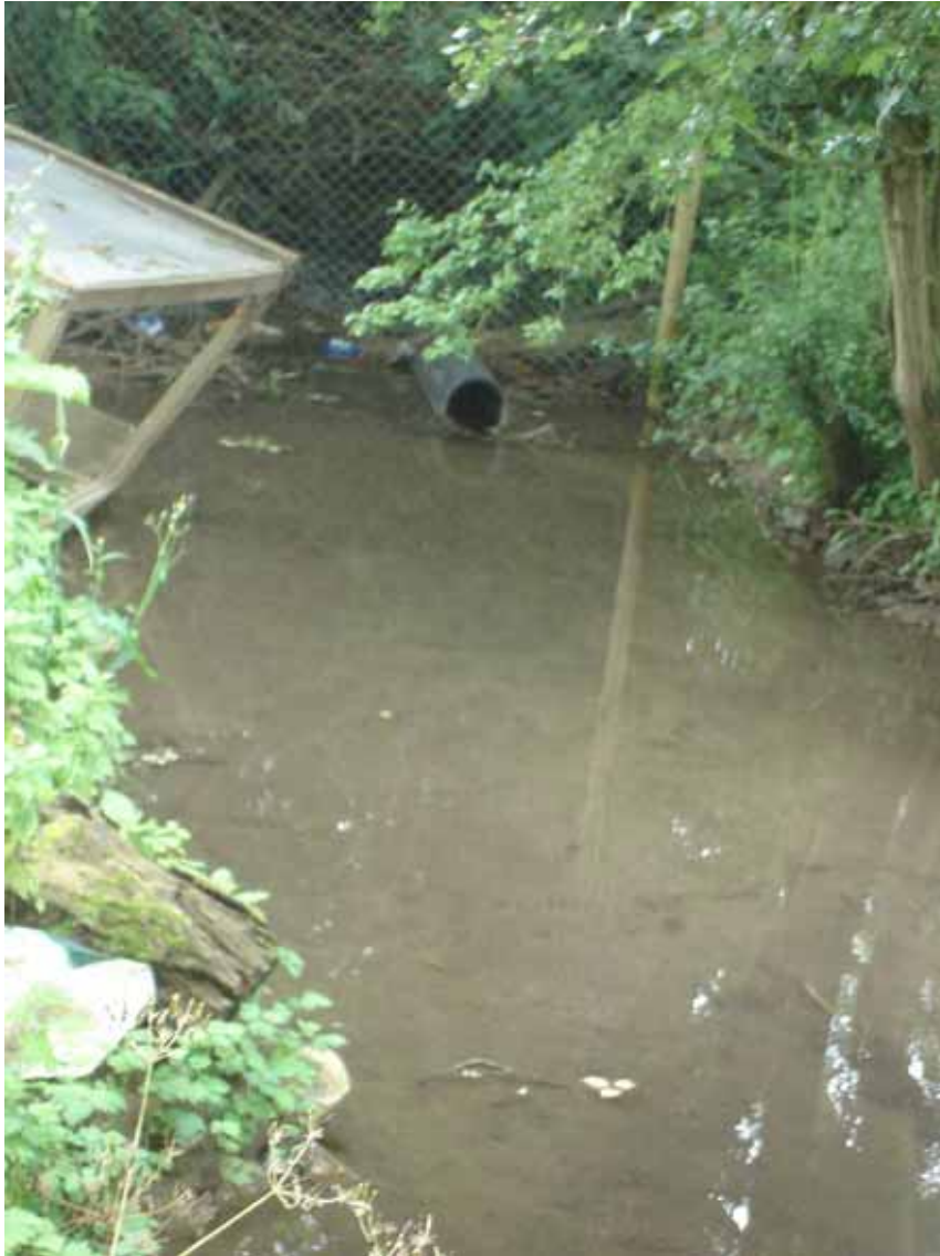
Area 2 – open watercourse adjacent to sewage works
