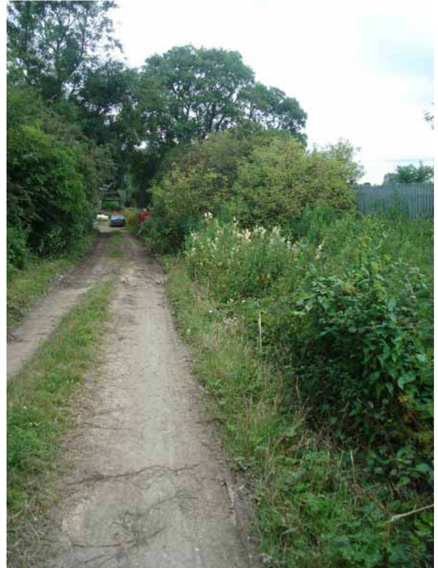
Area 2 – blocked watercourse leading to River Windrush
