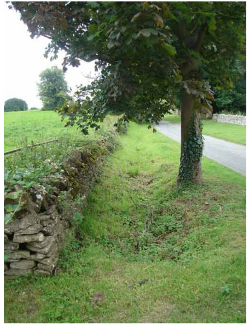
Area 1 – Ditch on south side of Westhall Hill that needs reforming
