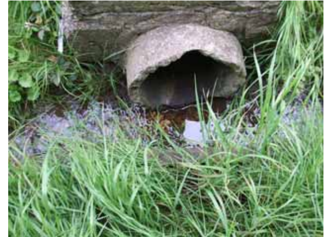
Area 1 – Culvert under Witney Road west
