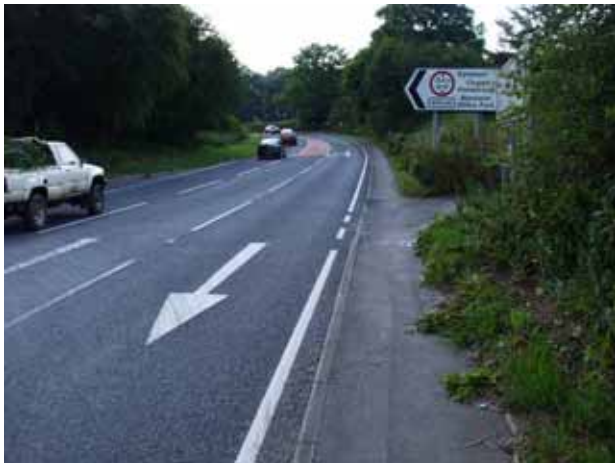
Area 4 – Junction with Lower Road
