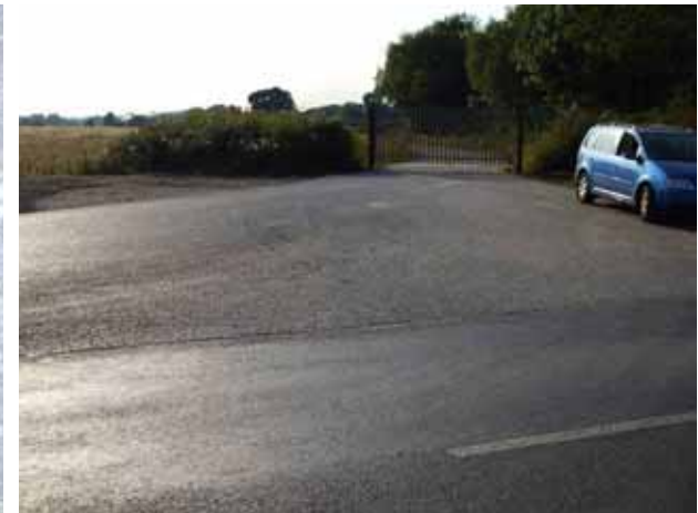
Area 4 – Entrance to Landfill Site
