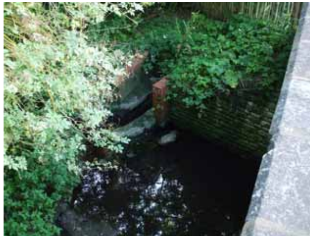
Area 4 – Highway drain into culvert at junction
