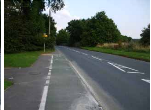
Area 3 – West of Witney Road, Railway bridge
