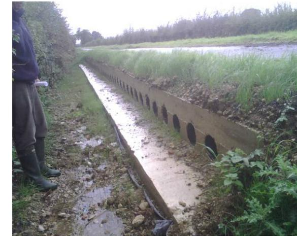
New multi-pipe flood relief structure, installed by OCC (downstream side) - 05/09/08
