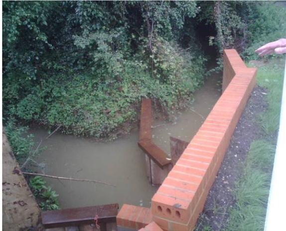
Upstream side of culvert, rebuilt by OCC since July '07 (note driven steel piles directing flow) – 05/09/08
