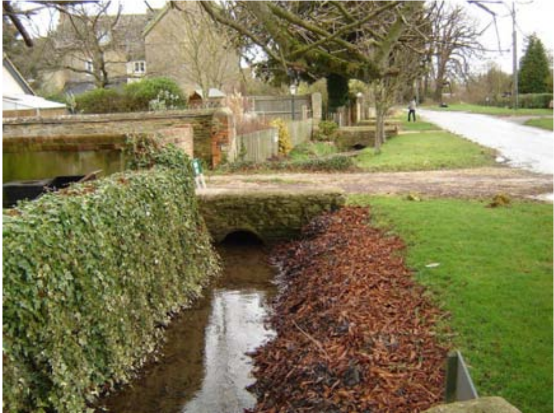
Area 2 – Northmoor Village Village brookcourse requiring upsizing of crossing culverts
