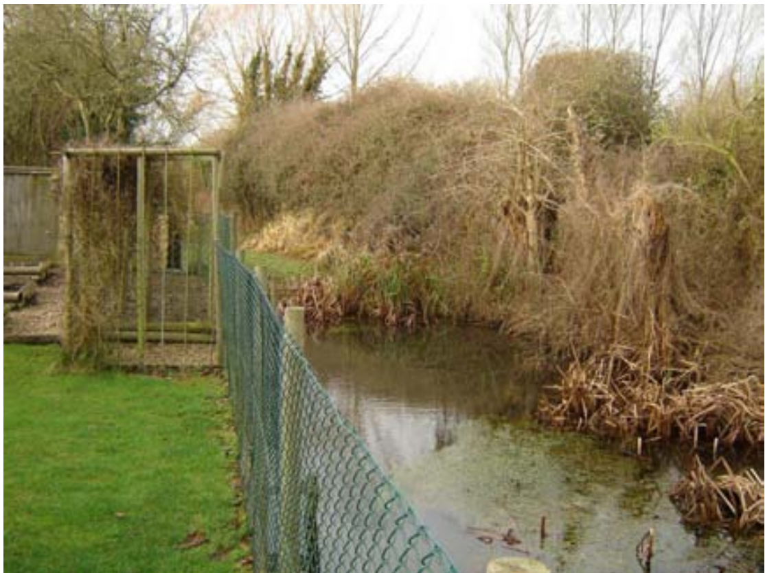
Area 2 – Northmoor Village Overgrown village brookcourse at “The Patch” requiring cleaning out
