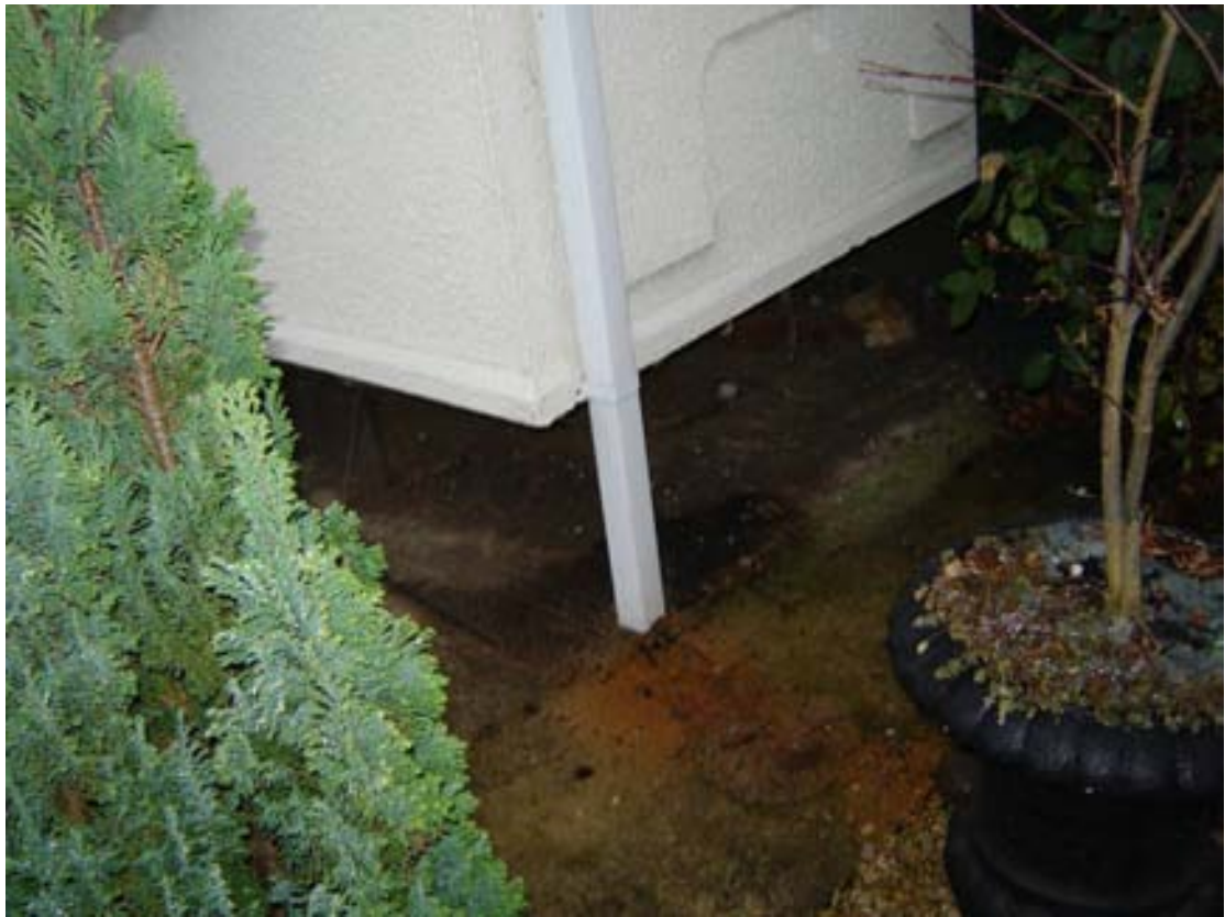
Area 1 – Bablock Hythe Flooded caravan at Thameside Caravan Park to be raised by 300mm
