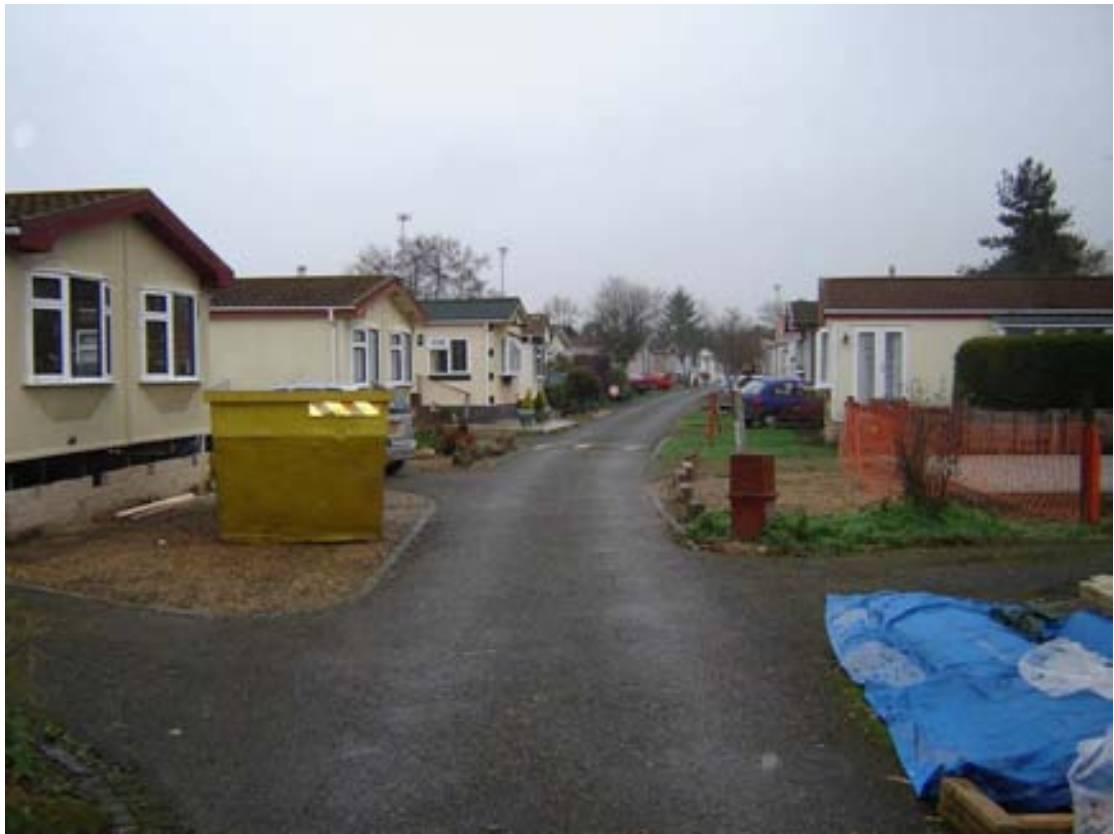
Area I – Bablock Hythe Thameside Caravan Park undergoing flood improvement works
