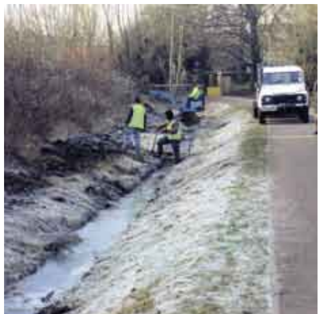
...The Council's Ditch Clearing Team working on the same ditch.
