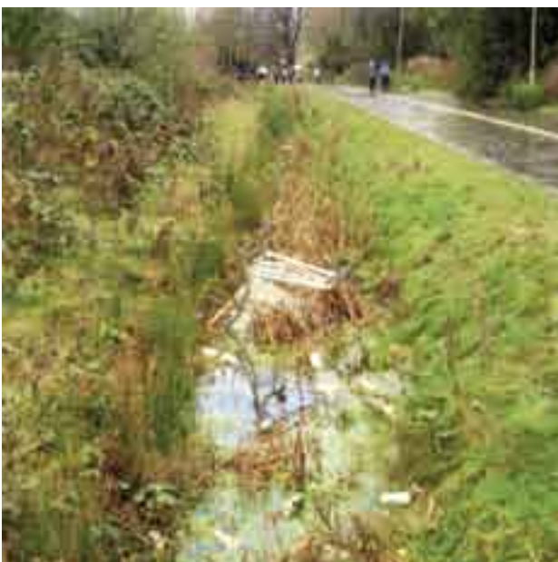
The over-grown ditch near Henry Box School, Witney before being cleared...
