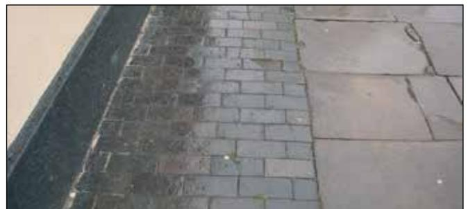
Traditional vehicle crossover surfaced with an irregular grid of stone setts; and a modern interpretation using concrete block paviours.
