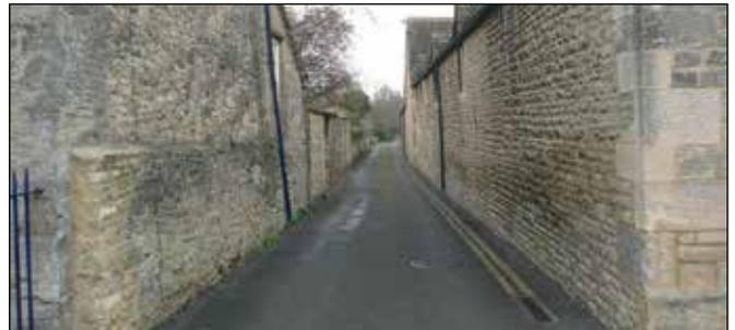
Simple pedestrian/ cycle route with informal alignment and landscaped edges: the surface is bituminous with embedded aggregate.
