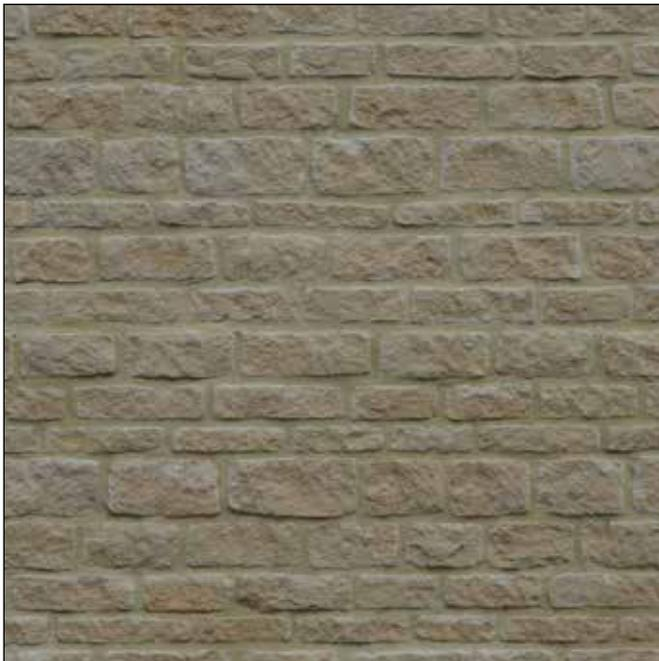
Fig. 8 Artificial stone wall
