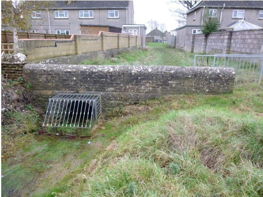
Figure 7 - Photo of Hailey Road drain culvert inlet showing installed trash screen and removed section of headwall
