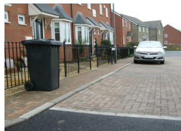
Pavers must be able to withstand the weight of collection vehicles; drop kerbs assist the movement of bins
