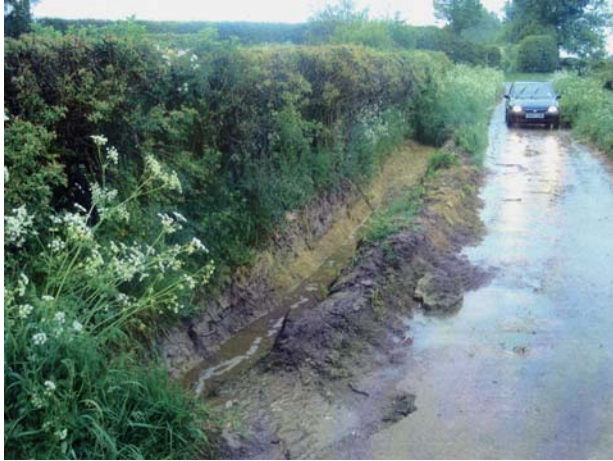
Area 3 - Cling Clang Lane, upstream side
