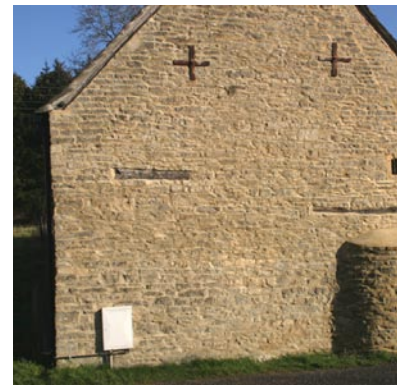
Fig. 1 Local limestone walling
