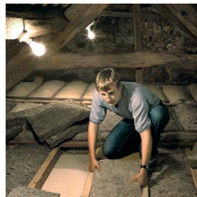
Fig. 14 Insulation laid between joists
