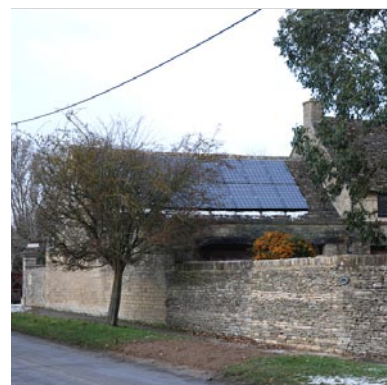
Fig. 29 Visually prominent photovoltaic panels on traditional building
