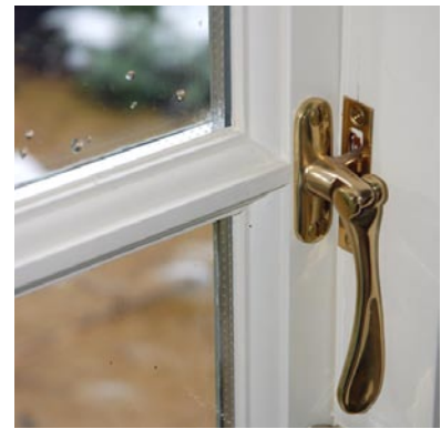
Fig. 18 Slim double-glazed units with well detailed glazing bars
