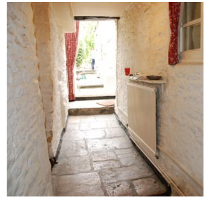
Fig. 3 Traditional stone slab flooring
