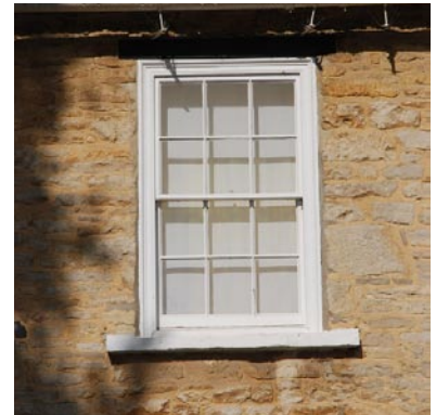
Fig. 10 Vertical sash window
