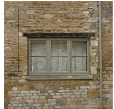
Fig. 9 Flush casement windows
