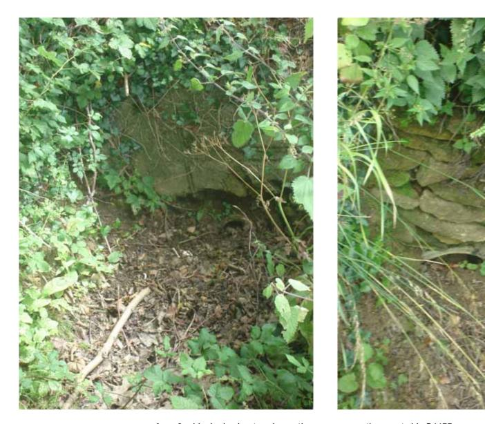
Area 2 – blocked culvert underneath access on north – west side B4477
