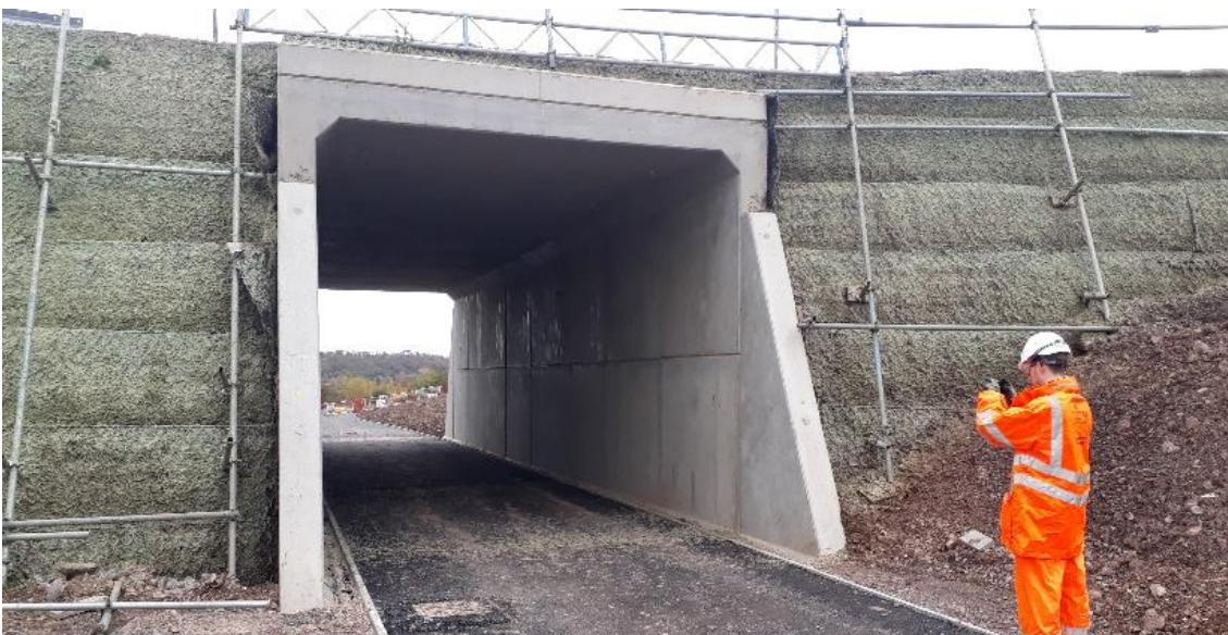
Figure 6.3: A pre-cast concrete subway nearing completion, 4m wide and 4m high
