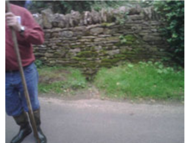
Highway drainage outlet at a Church Enstone Road culvert.
