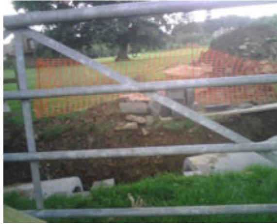
Works in progress on ordinary watercourse in land of Cherwell House
