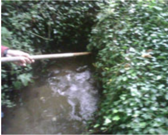
Outfall of culvert in grounds of No Oven House
