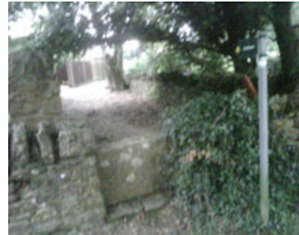
Public footpath on Chipping Norton Road. Fall of footpath is towards Chipping Norton Road.
