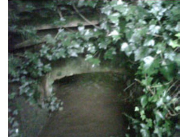
Footbridge at rear of No Oven House on watercourse
