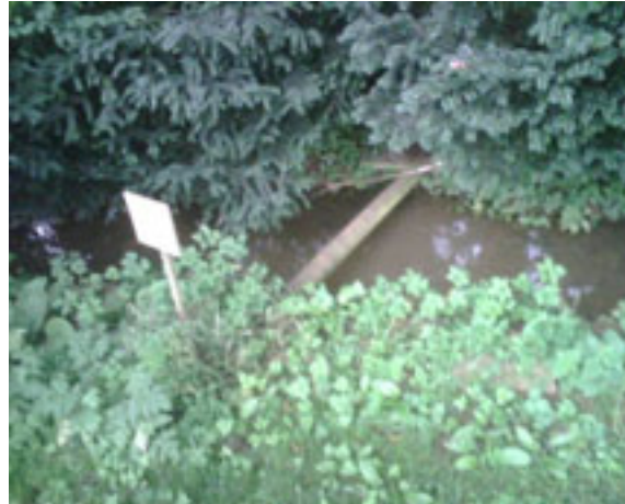
Remains of footbridge support at rear of No Oven House
