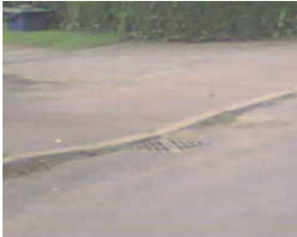
Dropped kerbs at entrance way to Chapel Lane
