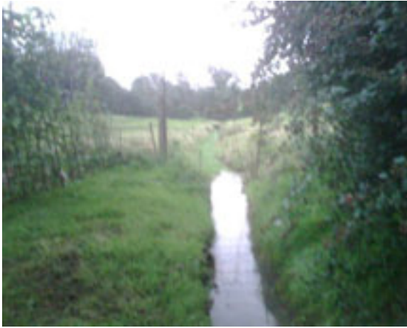
Watercourse at rear of Chapel Lane, looking downstream
