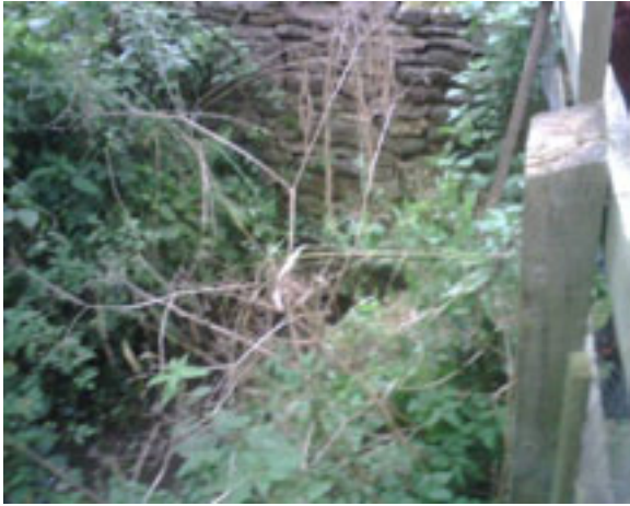
Outfall on culvert on Church Enstone Road
