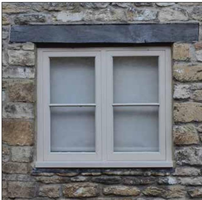
Fig. 1 New traditional flush, side-hung casement window
