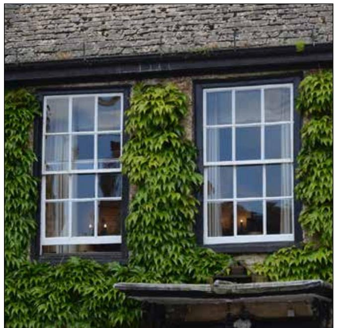
Fig. 2 Traditional vertical sliding sash windows
