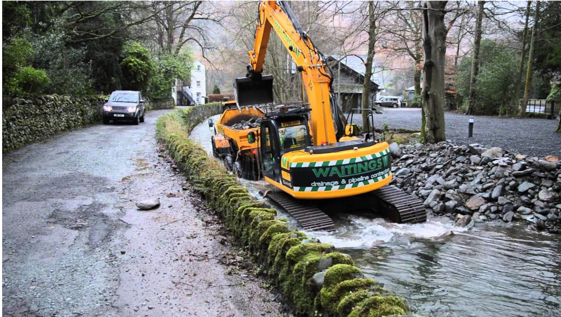
Wide Track Excavator Working in channel With Dumper Truck
