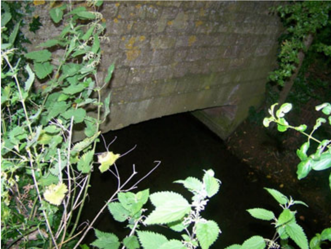
Broadwell Brook at Broadwell Road – very low soffit
