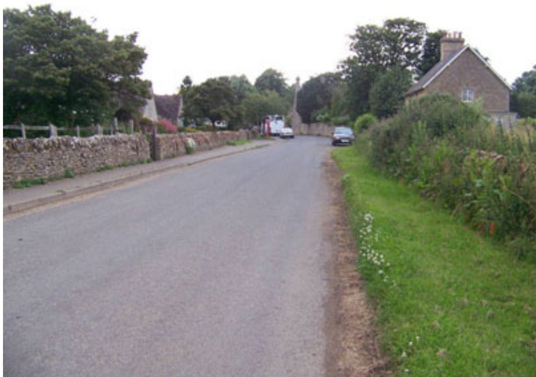
Filkins Road – Church Row Cottages on left, very flat – wall and higher ground on right which traps water
