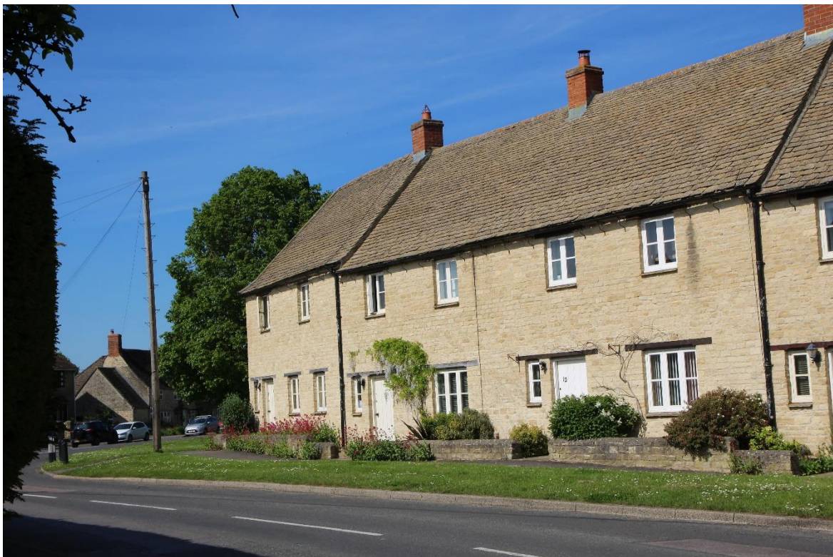
Figure 16. Modern development in the village Conservation Area stated as being in keeping with the vernacular style of the village. Note the use of similar materials to traditional cottages in the village centre including stonework and roofing material.
