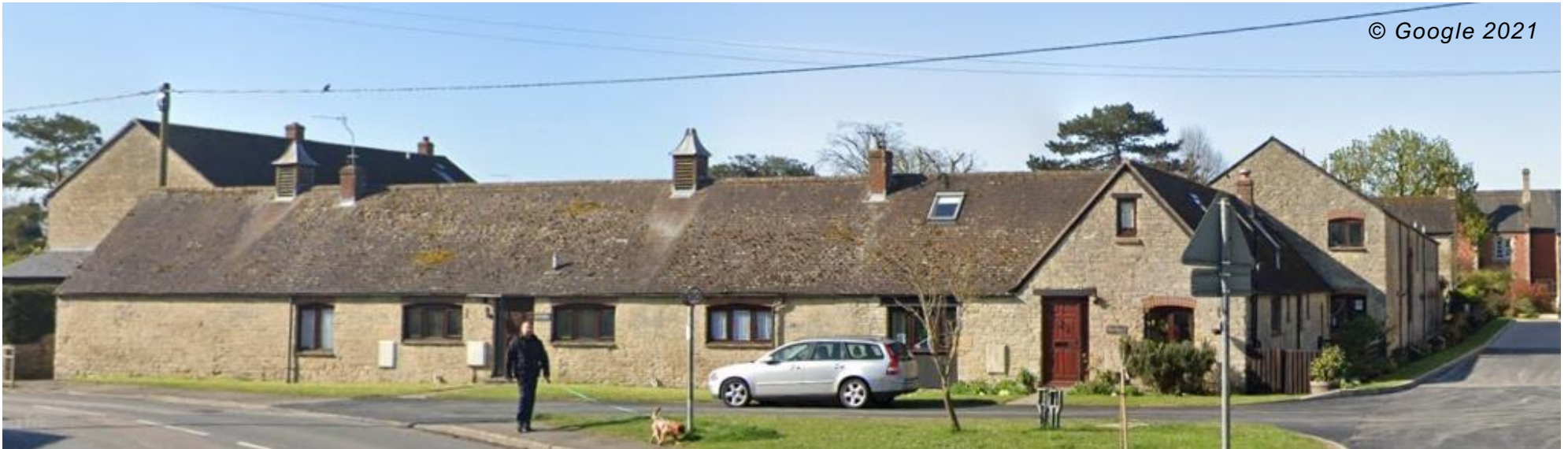
4-8 Hollow Furlong, Wild Forest and The Old Stables Former barn buildings converted as part of cul-de-sac development in 1980s.
