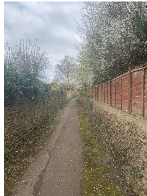
Drystone walls in the walkway linking the Upper and Lower Greens
