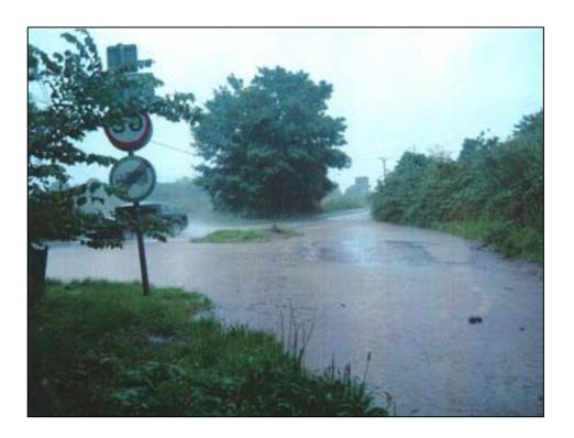
Photo 4 – Kilkenny Lane at junction with Burford Road, illustrating poor highway drainage
