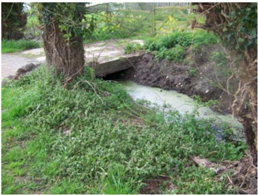
Minimal ditch capacity at Manor Farm – entire section requires deepening, minimal clearance under access bridge
