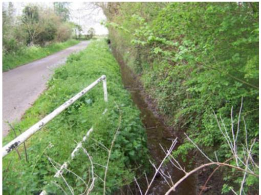
College Ditch looking east out of village from culvert under road. Note minimal ditch capacity in village
