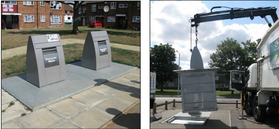
Figure 3: Left; image of two retrofitted URS with a low rise flat residential area in Peterborough City. Right; a crane operated waste truck pictured emptying of a 5,000l URS unit. A single waste collection worker is capable of operating the system.
